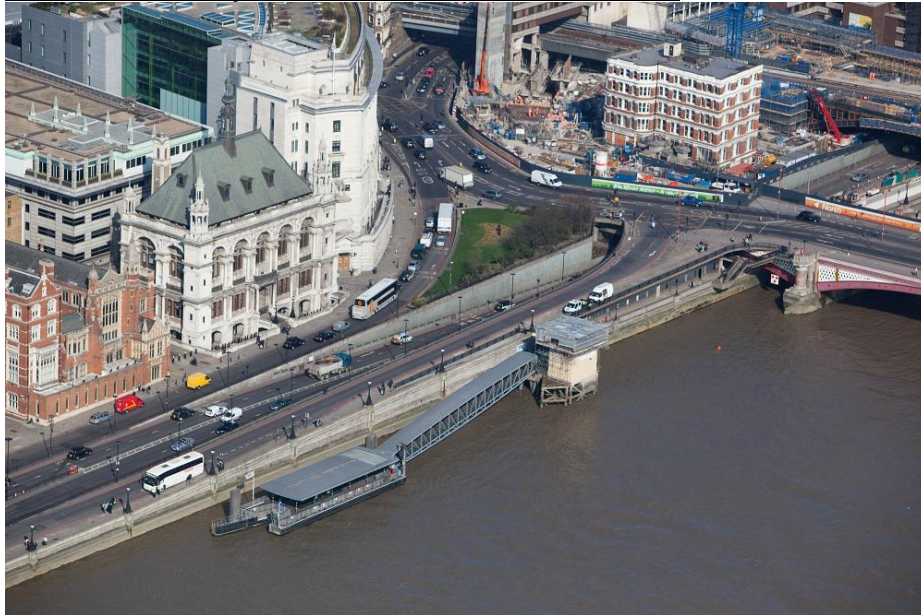
Thames Tideway Tunnel Location at Blackfriars
